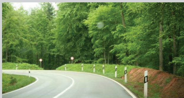
Picture 18 - Earth walls replacing guardrails
