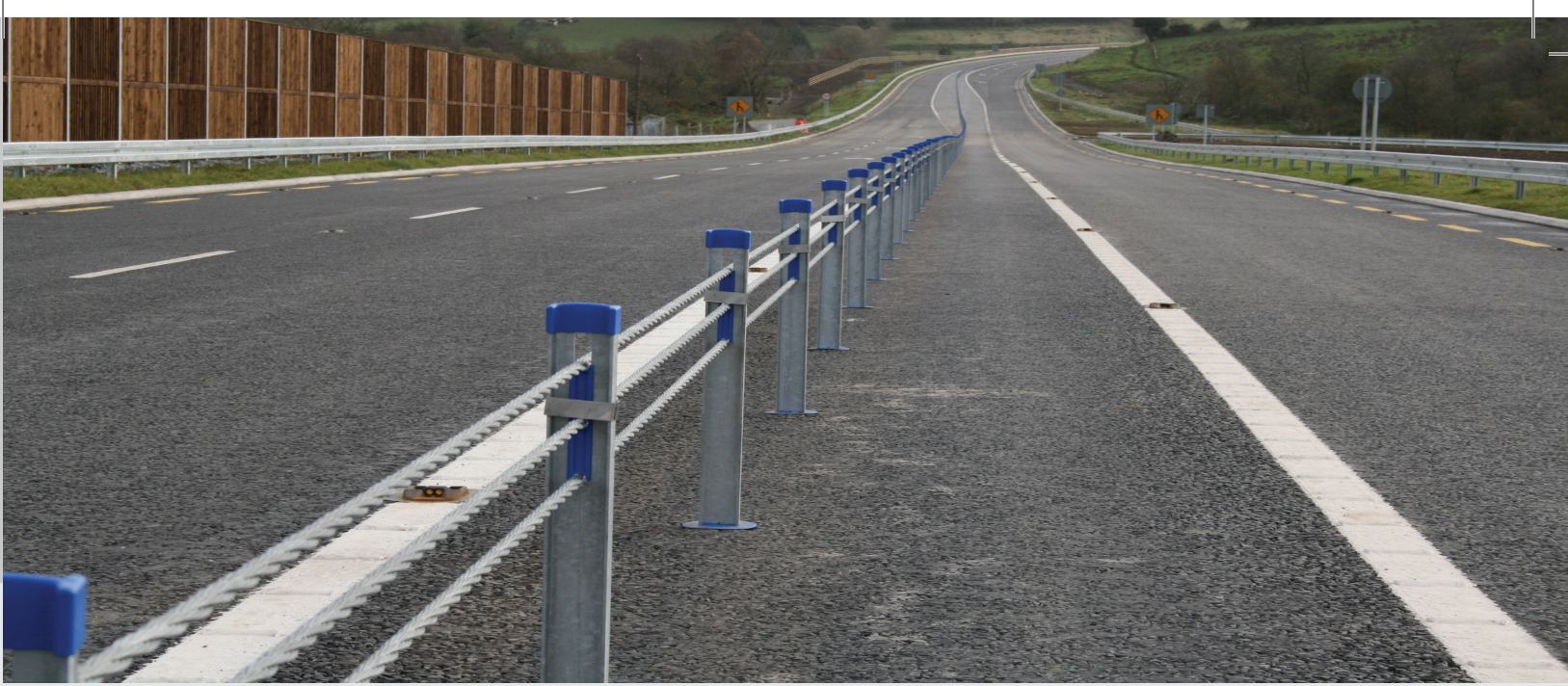
Picture 7 - Wire Rope Barrier
