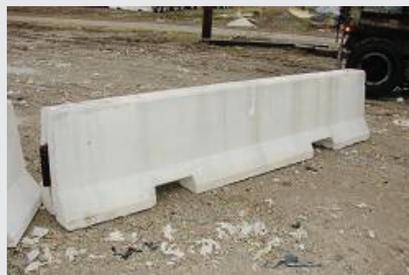
Picture 6 – Pre fabricated concrete barrier
