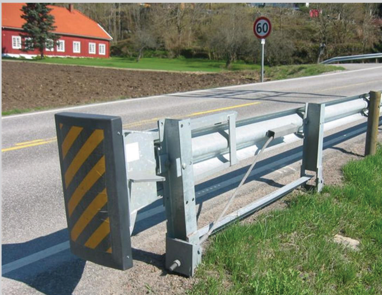
Picture 26 - Guardrail terminals present sharp edges and a low contact surface, face traffic directly and are located very close to the roadway. Fitting them with a protective cover reduces the risk of injury on impact.
