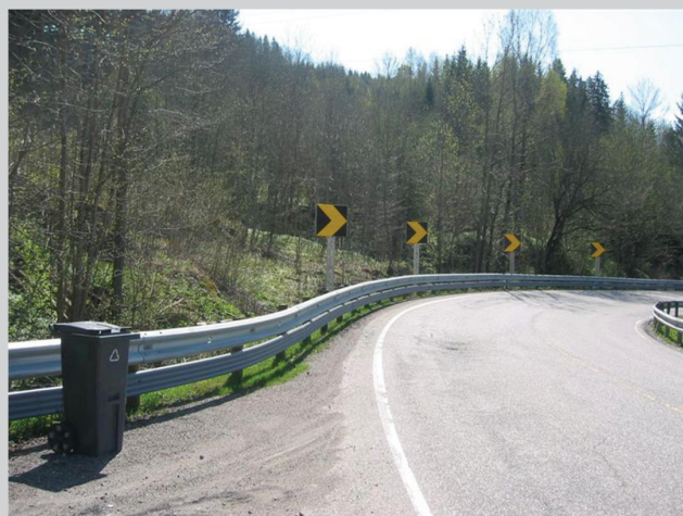
Picture 24 - Here signposts have been placed behind a guardrail equipped with MPS.
