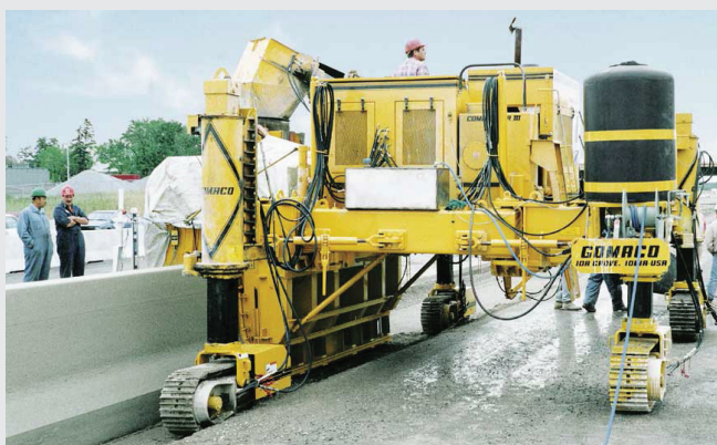
Picture 5 - Slip formed concrete barrier
