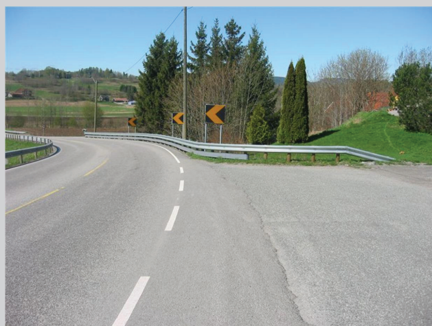
Picture 25 - Dangerous terminals have been replaced with MPS swinging away from the roadway.
