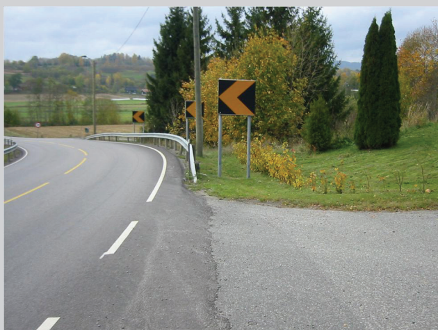
Picture 25 - Dangerous terminals have been replaced with MPS swinging away from the roadway.
